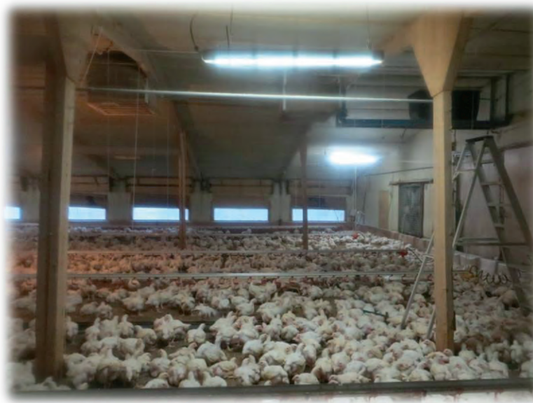
Figure 21 shows a fluorescent light which is facing the wrong way, potentially allowing air coming in through the inlets to hit the light and fall to the litter
