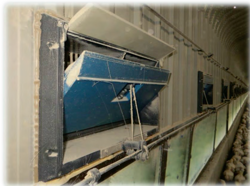
Figure 23 Recessed inlet at a farm in Devon (it also has a small deflector ramp to guide air up towards the ceiling)
